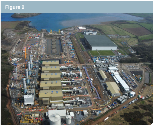
Pembroke Power Station with the intake and Pennar Gut in the background
