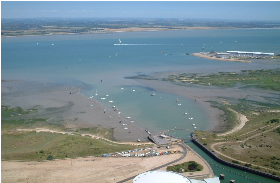
Figure 6-12 Fawley Power Station CW intake at low tide, showing the onshore CW inlet channel and bordering saltmarsh areas
