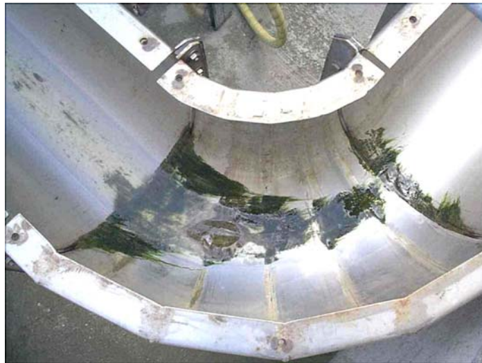
Plate 3.8 A sharp bend in this fish return gully demonstrates the issue of biofouling where uneven joints have encouraged algal growth, causing a flatfish to take cover there. A smooth surface or exclusion of light would have prevented this.
