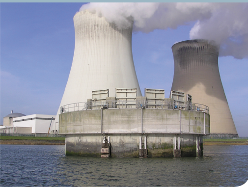
Acoustic Fish Deflection System deployed on Doel 3&4 Cooling Water Intake
