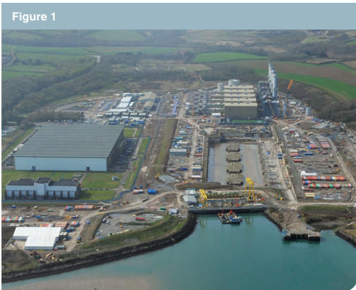
Pembroke Power Station with the intake in the foreground
