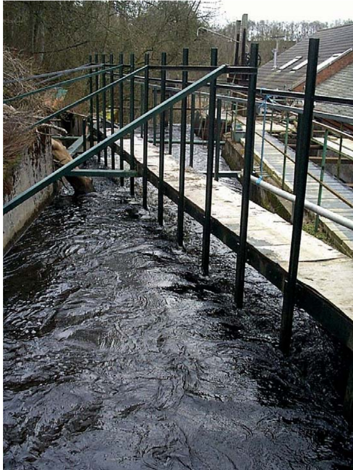
Plate 3.11 The louvre screen at Almond Bank Power Station. Only the superstructure is visible.
