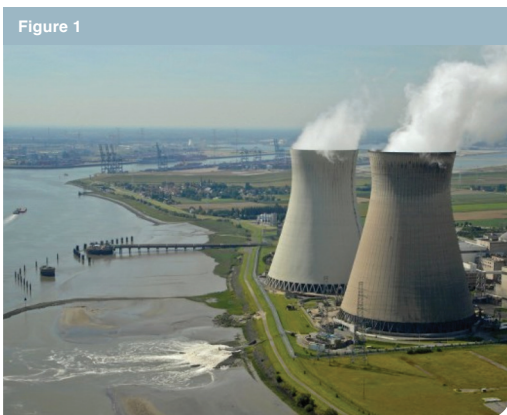
Water Intakes and Outfall at Doel Nuclear Power Plant, Belgium
