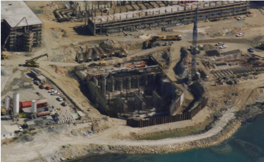
Figure 4-8 CW pumphouse substructure under construction at Vasilikos, Cyprus
